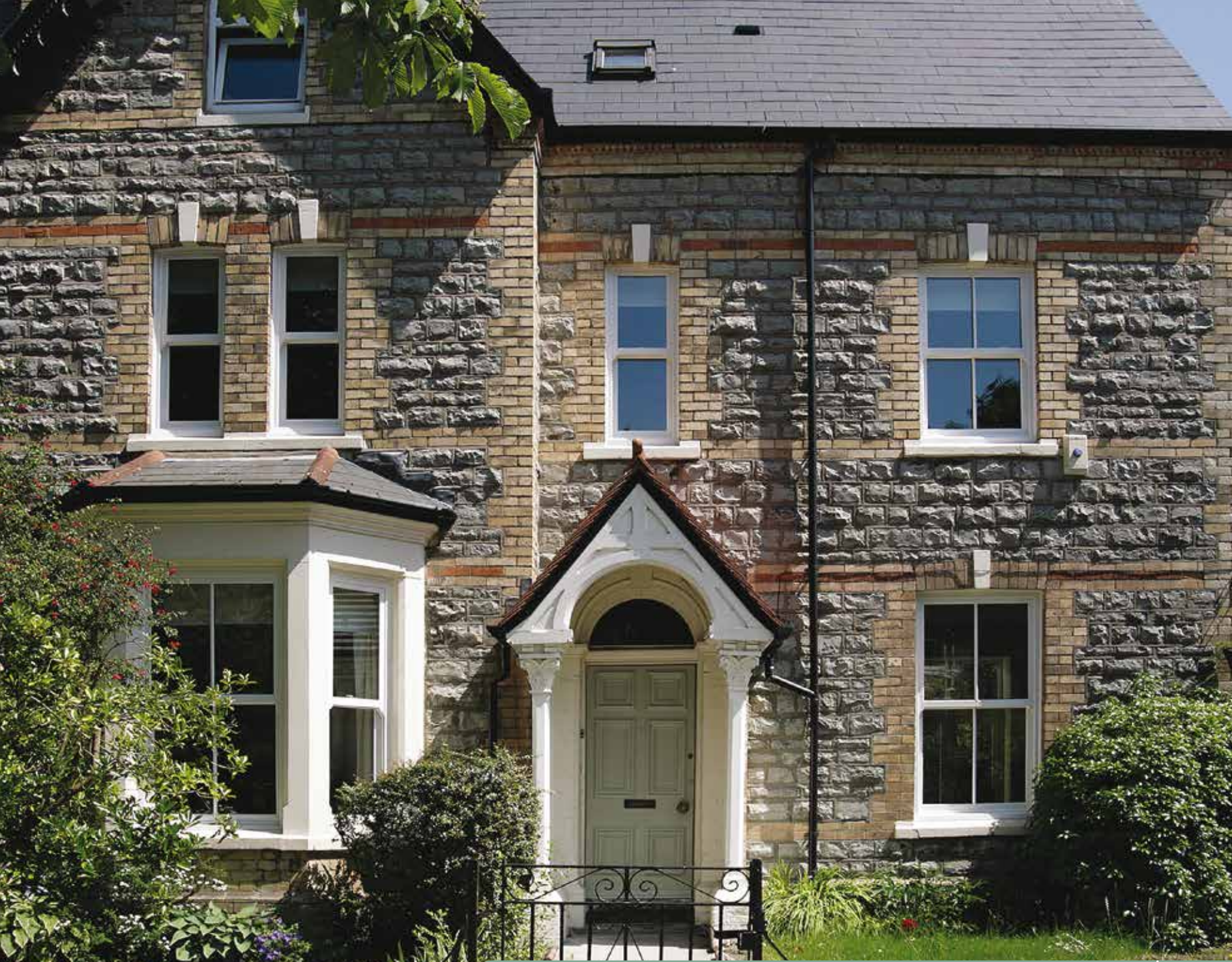
Vertical sliding sash windows with decorative horns and single Georgian bar ▲
